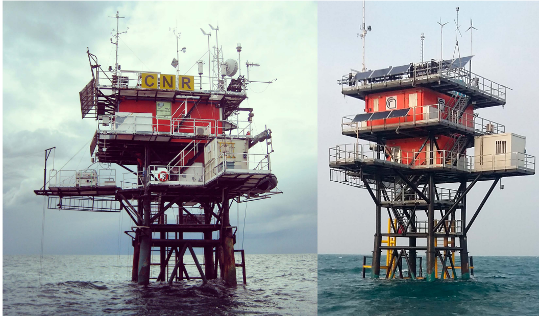
FIG. 3. The ISMAR oceanographic tower Acqua Alta. (left) The original structure used during the measurements; (right) after the restoration in 2018. The emerged working part is now 2 m higher. See Fig. 2 for its position.
