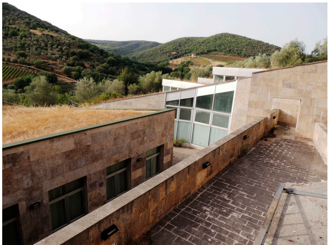
Figure 22. The Tabor reception centre near Castelnuovo dell'Abate, where the cladding of the walls has been realized with travertine from the nearby quarries (credit Silvia Rescic).
