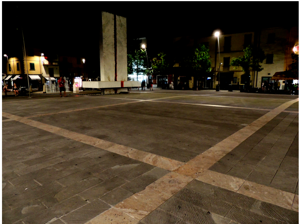
Figure 21. The paving of Risorgimento square in Quarrata (Pistoia), realized with a decoration of travertine light-coloured bands in contrast to the grey of the Pietra Serena sandstone (credit Silvia Rescic).
