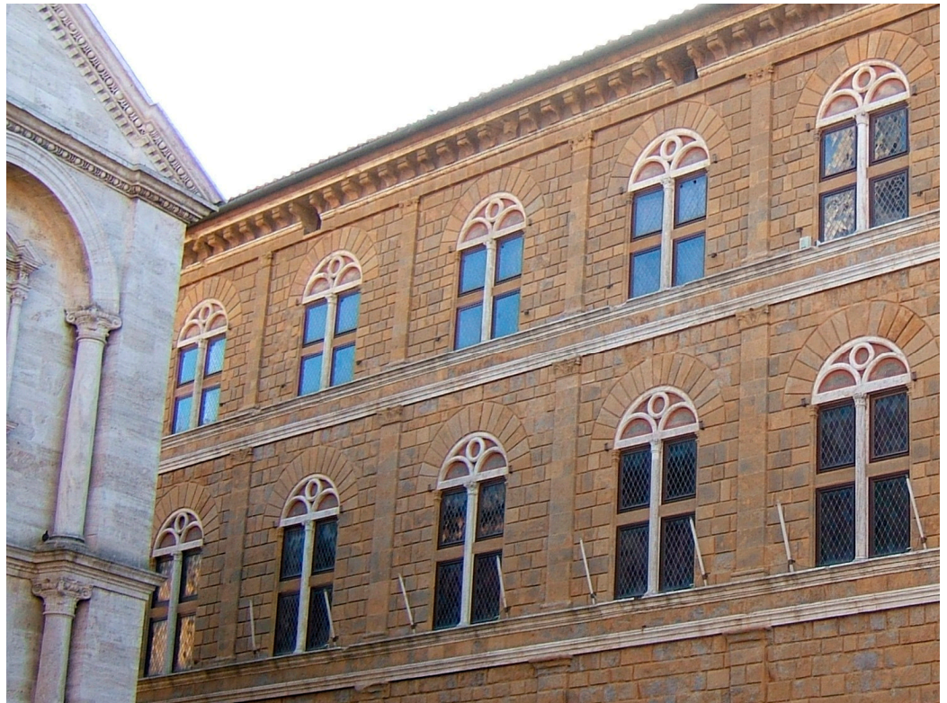
Figure 9. Pienza, Palazzo Piccolomini (XVth century), with the façade in finely hewn Pliocene sandstone and window frames in travertine. On the left, part of the Cathedral façade can be seen, with its travertine cladding (credit Barbara Sacchi).
