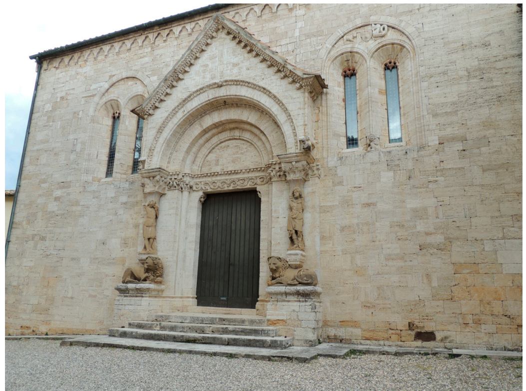
Figure 5. The finely hewn ashlars of the Church of Santi Quirico and Giuditta (XIIth–XIIIth century) in San Quirico d'Orcia (province of Siena). The portal is surmounted by a porch supported by caryatids resting on lions made of Pliocenic sandstone (credit Barbara Sacchi).
