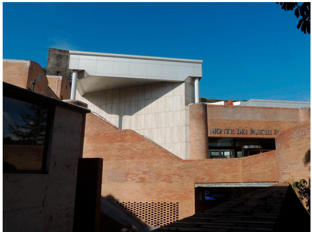
Figure 19. The new Monte dei Paschi di Siena bank business centre with the use of bricks and Rapolano travertine cladding (credit Silvia Rescic).
