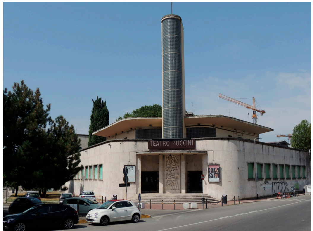
Figure 15. The socialization spaces (now transformed into a cinema) of the Manifattura Tabacchi in Florence (credit Fabio Fratini).
