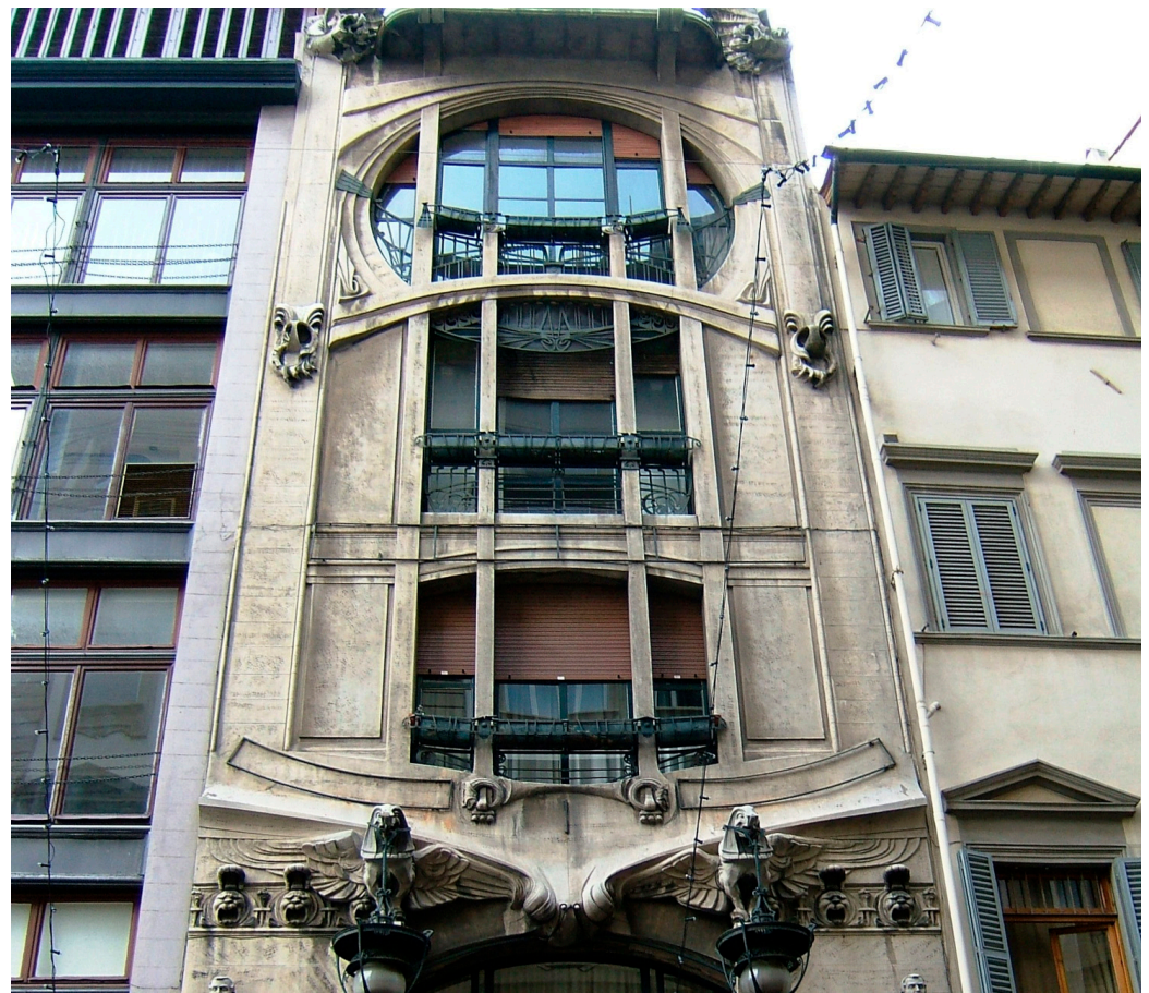
Figure 18. The Casa-Galleria Vichi in Florence, an Art Nouveau building with a cladding in artificial travertine (credit Fabio Fratini).
