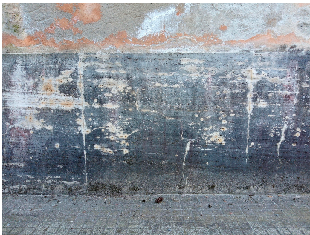
Figure 23. Dark-grey biological colonization and predominantly clay-size mineral particles deposition in a travertine baseboard (credit Oana Adriana Cuzman).
