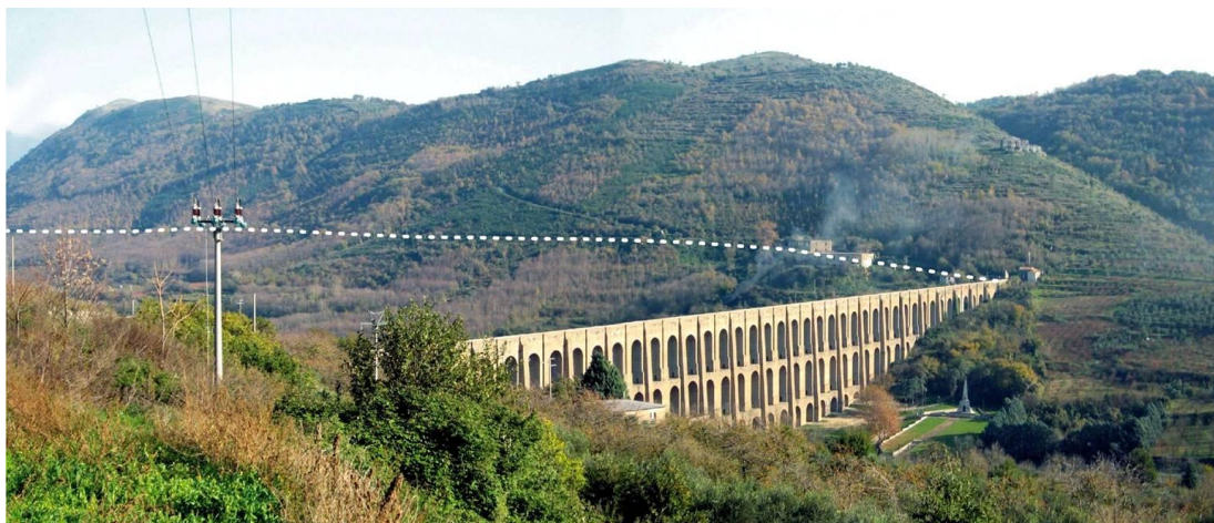
Figure 2. The Carolino aqueduct (Campania, Italy): the white dotted line marks the underground development (photo courtesy S. Del Prete).
