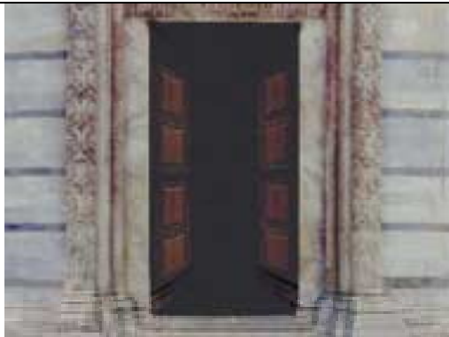
Picture 3: The open portal (photo).
