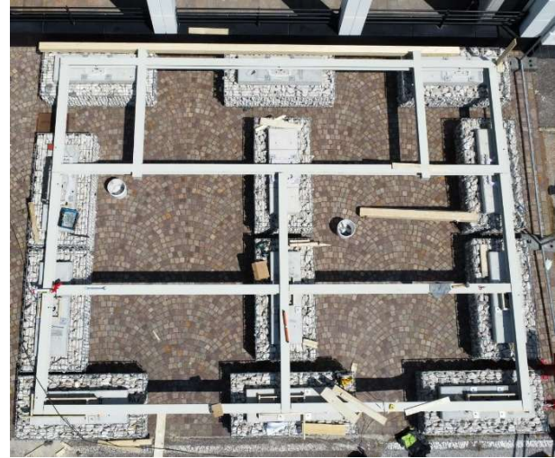
Figure 3. Example of connection between orthogonal capping beams (left) and LSF system (right)
