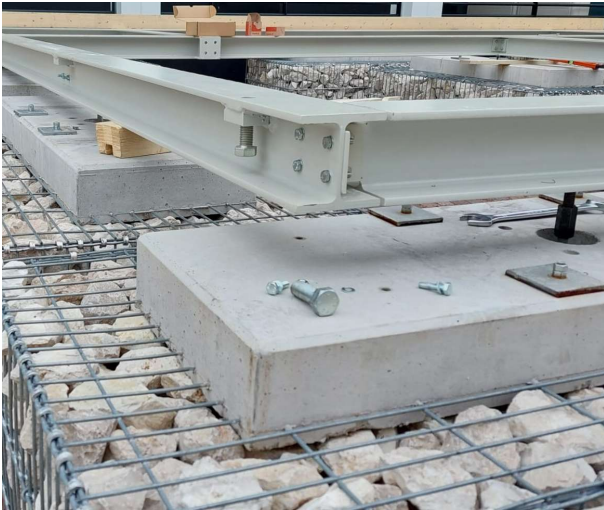
Figure 3. Example of connection between orthogonal capping beams (left) and LSF system (right)
