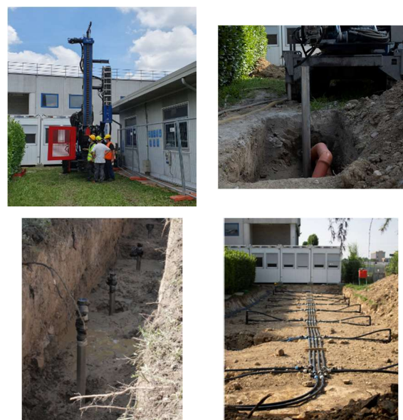
Figure 3: Pictures from BHE field at CNR pilot site in Padova.
