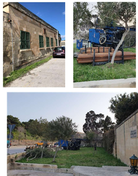
Figure 10: Site and drilling for BHE in Valetta demonstration project.
