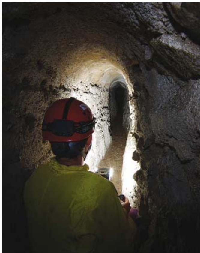
Fig. 1 - Within a branch of the underground aqueduct, dating back to XIX century, at Montecompatri, Latium (photo archive Egeria Centro Ricerche Sotterranee).
