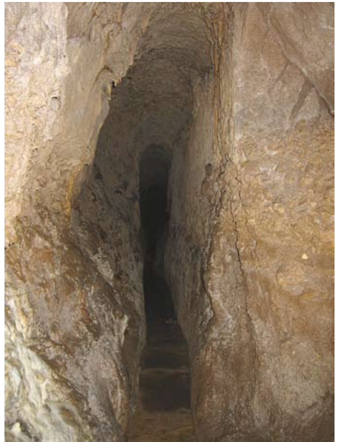
Fig. 7 - Roman aqueduct at S. Egidio del Monte Albino (Campania; photo S. Del Prete). The picture shows development of calcite deposits in a sector of the hydraulic work dug in fan gravels alternating with pyroclastic deposits.
