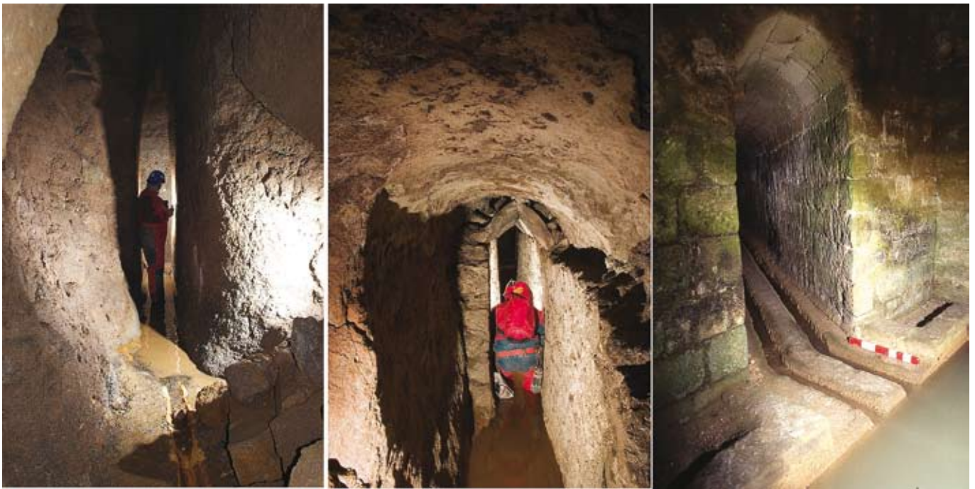
Fig. 5 - Examples of underground aqueducts: a) ancient aqueduct, re-worked in the XVII century by monks of the Camaldoli Hermitage at Mount Tuscolo (Latium); photo archive Egeria Centro Ricerche Sotterranee; b) branch of the late roman aqueduct at Roccarainola (Campania), realized in pyroclastic deposits; photo F. Maurano; c) channels within the aqueduct Fontana della Stella at Gravina in Puglia (Apulia); photo G. Bologna.
