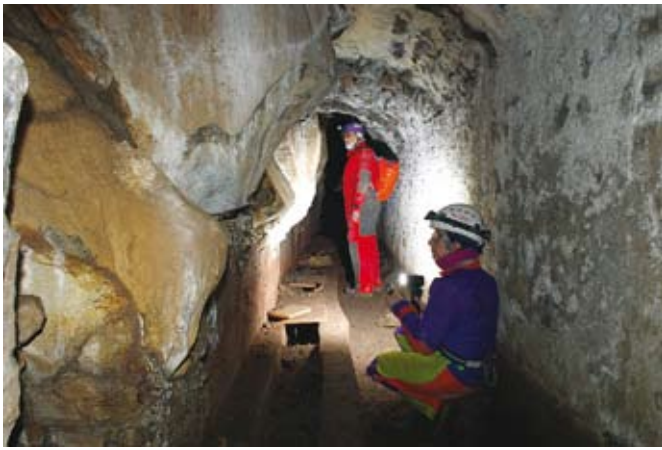
Fig. 6 - Covered channel on one side of the gallery at the Montecompatri aqueduct, Latium (photo archive Egeria Centro Ricerche Sotterranee).
