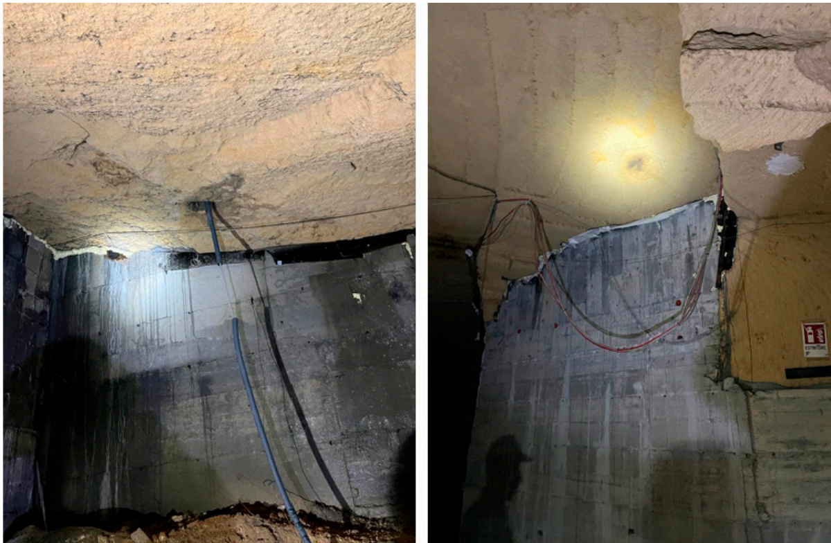
Figure 25. Photos of the consolidation interventions.
