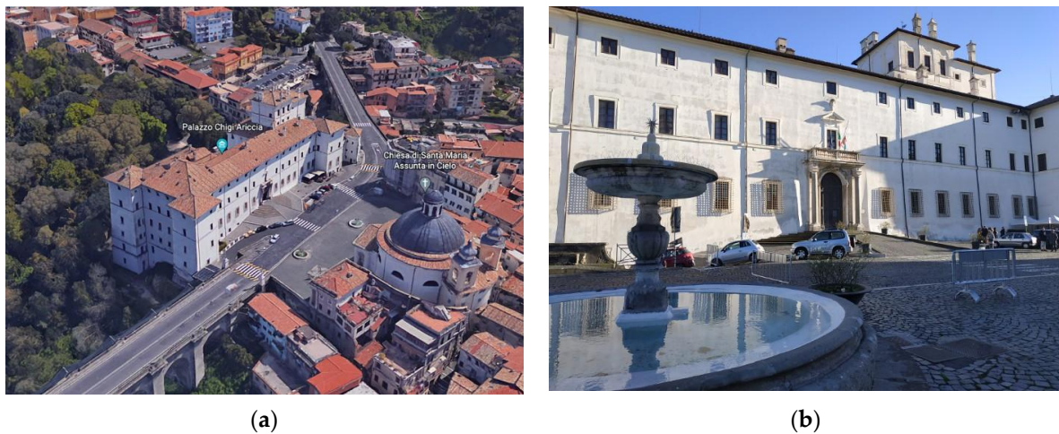
Figure 1. (a) Aerial view of Ariccia by Google Earth showing the Chigi Palace from the left side; (b) front view of the Chigi Palace from Court Square (Piazza di Corte).
