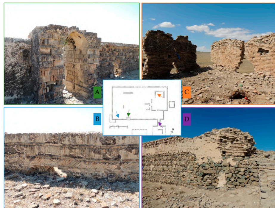
Figure 2. Photos of the palace ruins taken during the sampling campaign in 2017 showing the remains of the perimetral walls and their building technique. Coloured arrows in the central map represent the photo shooting points: (A) one of the doors at the South wall, (B) particular of the building technique of the bricks masonry at the South wall, (C) remains of interior brick masonries at the north-east side of the ruins and (D) remains of the masonries built with stone and bricks and partially covered by plaster located at south-east gate of the palace.
