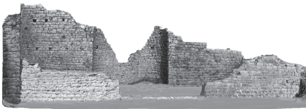
Fig. 10 3D digital model of the east-west front of the Doclea forum , obtained by a laser scanner survey ( after RINALDI TUFİ, BARATIN, PELOSO 2010, fig. 6).
