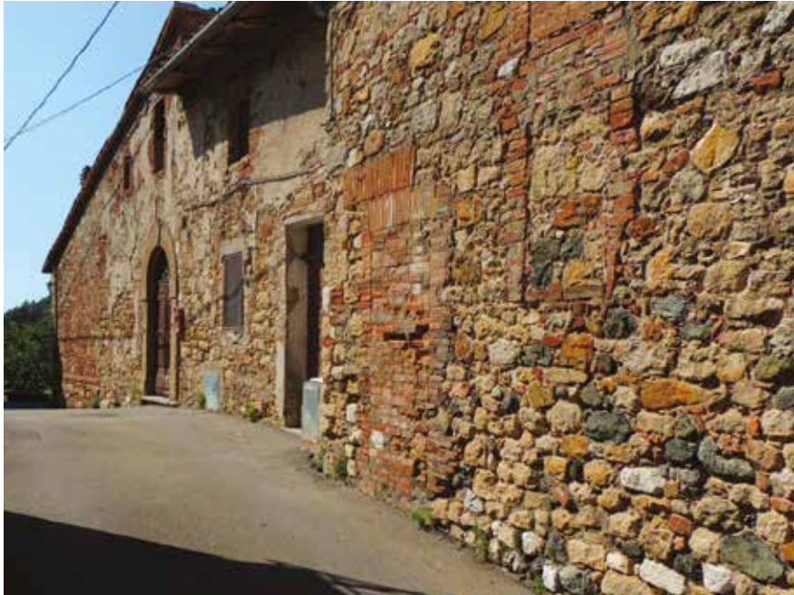
Fig. 8 Montecastelli: mixed masonries made of unshaped/ roughly shaped blocks made of prevailing organogenic limestone and bricks, serpentinite, marly limestones.
