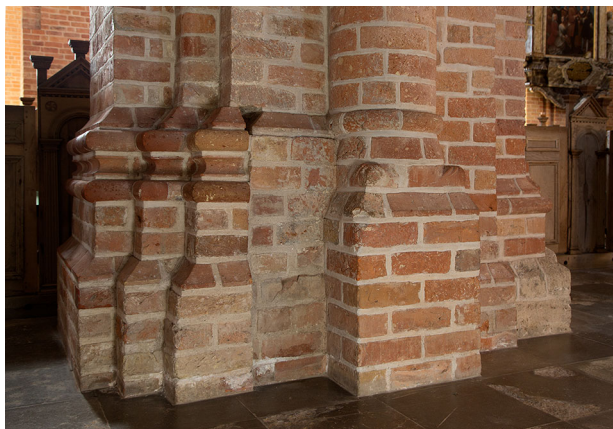
Fig. 18 | Column in Ringsted Cathedral. The groves are wide, up to 2 centimetres. Not all angles are 90 degrees (Photo: Thomas Olsen).
