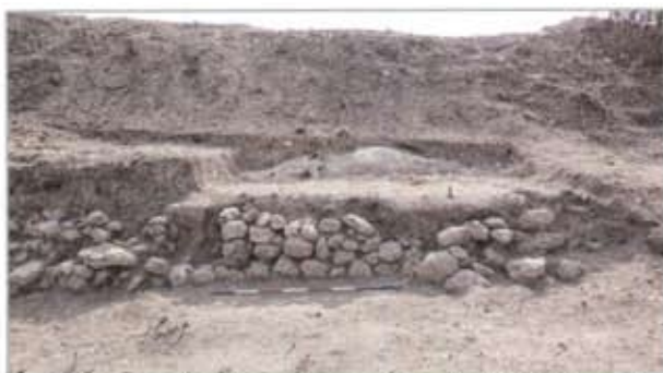
Fig. 6- Terrace wall of the western slope (photo by S. Festuccia).
