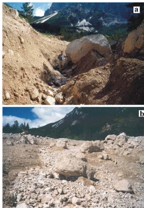
Fig. 4 Large boulders in the lower channel reach (a) and in the retention basin (b)
