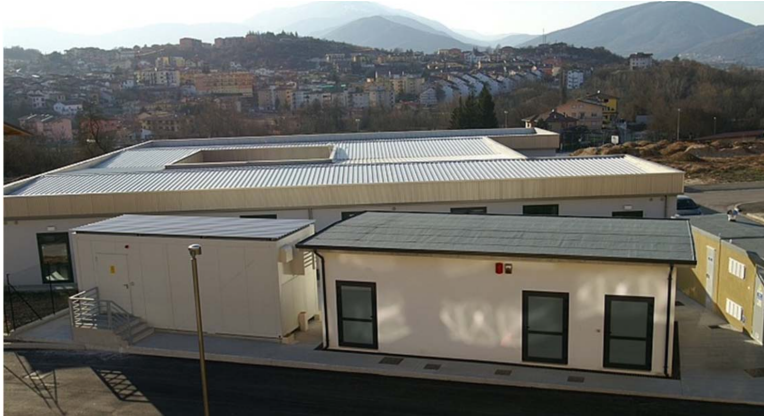
Figure YY: Univaq's shelter infrastructure
