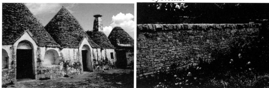
Figure 3. Rural architecture in Apulia: trulli (left), a typical countryside house, and dry-stone walls (right).
