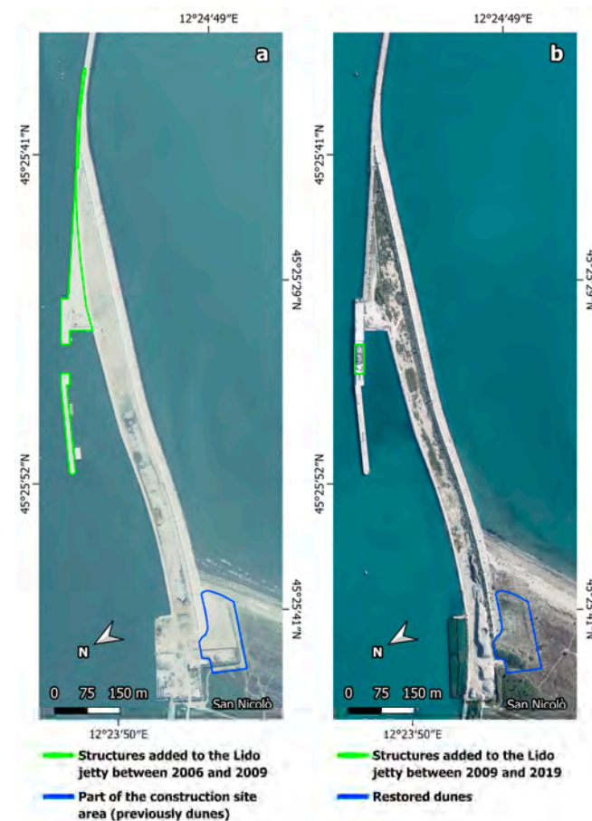
Figure 8. Coastal structures: (a,b) cell A, additional works at the jetty of Lido, including new structures (in green) at the northern edge of the island (aerial photographs taken in 2009; source: MAV).
