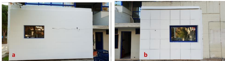
Figure 3. InnoWEE retrofitting: (a) ETICS-like panels in Office 1, (b) ventilated façade in Office 2 [source: InnoWEE project].
