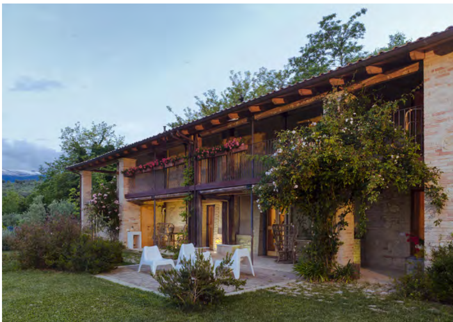
Fig. 6 Casalincontrada (Chieti) Borgocapo: earthen building (Fig. 5) after restoration
