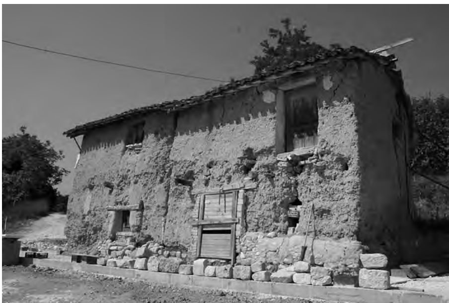
Fig. 5 Casalincontrada (Chieti) Borgocapo: earthen building before restoration
