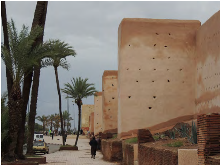
Fig. 11 The earthen plastered city walls of Marrakech
