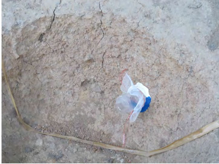
Fig. 9 In situ water vapour transmission test
