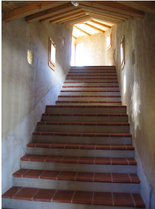
Fig. 4 Lightened earth wall with clay plaster in Panta Rei (by E. Baglioni, 2008)
