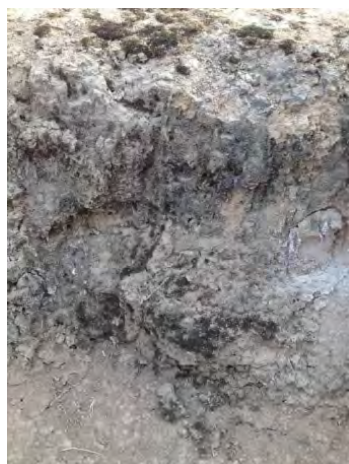
Fig. 3 Surface blackening in area F29 due to algae development
