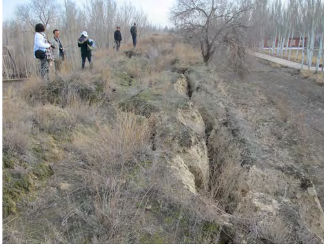
Fig. 5 Gully deterioration
