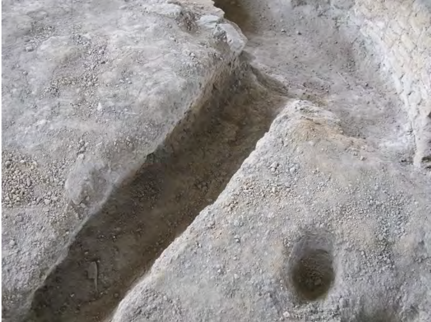
Fig. 2 Pulverization of the earth site: main phenomenon of surface decay
