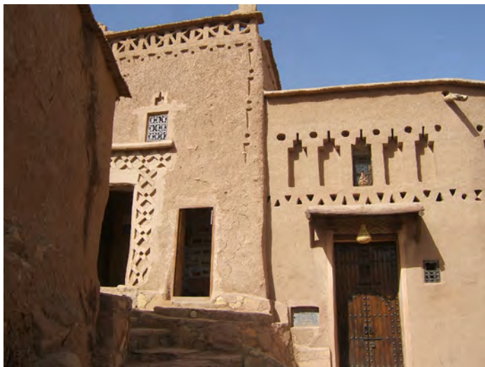
Fig. 5 Accurate maintenance of houses in the village of Ait Ben Haddou (Morocco)
