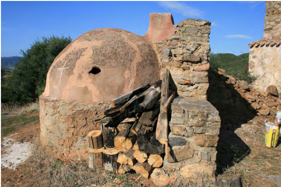
Fig. 8 Medau Tattinu de basciu, Nuxis (SU), raw earth oven during restoration (Photo Marco Bianchi)
