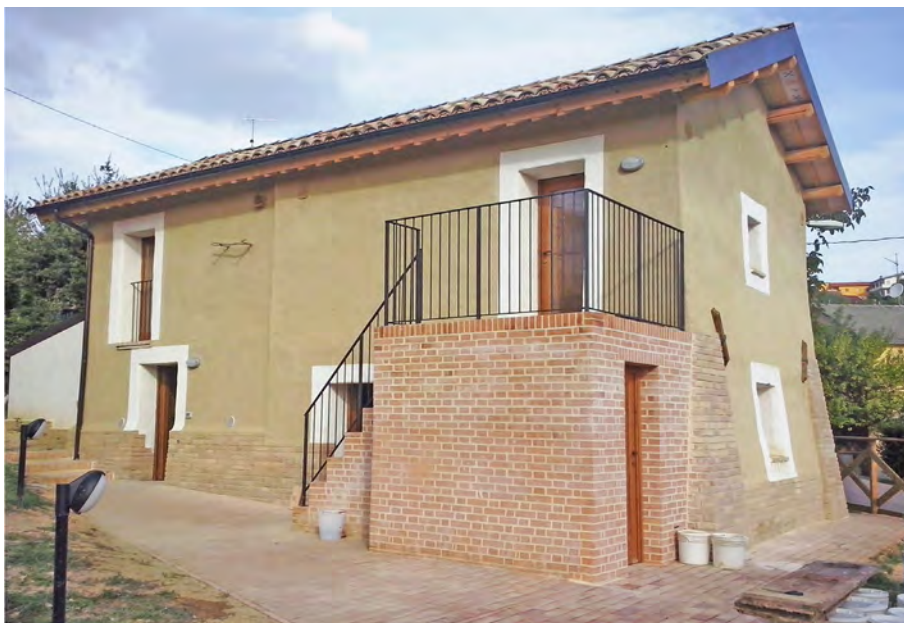
Fig. 10 Casalincontrada (Chieti): Teresa's house, after restoration
