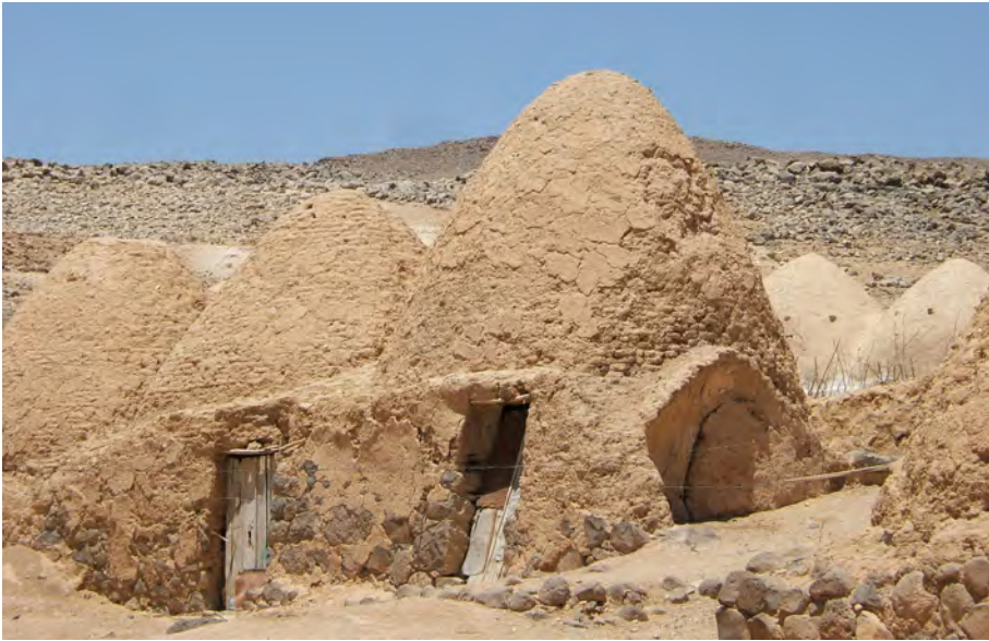
Fig. 3 Syrian corbelled dome house, lack of maintenance
