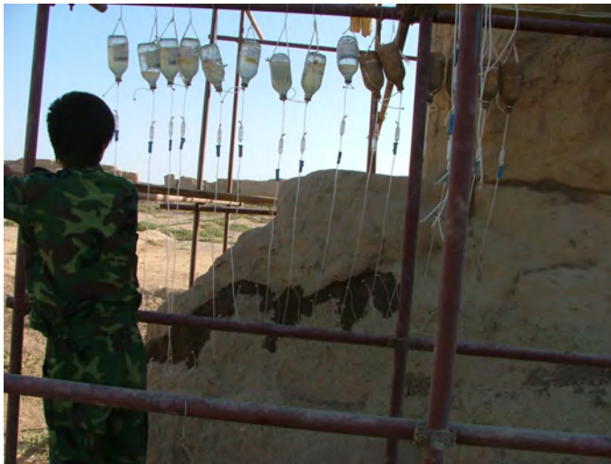
Fig. 11 Application of the consolidating product through dripping method
