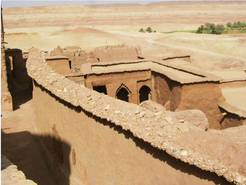
Fig. 9 Protection of the ridge of the walls to avoid water infiltration (Morocco)
