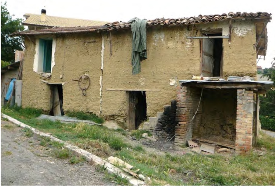
Fig. 7 Casalincontrada (Chieti): Teresa's house, before restoration
