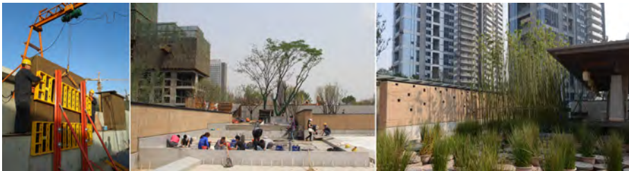
Fig. 12 Vanke landscape project based on developed rammed-earth technology
