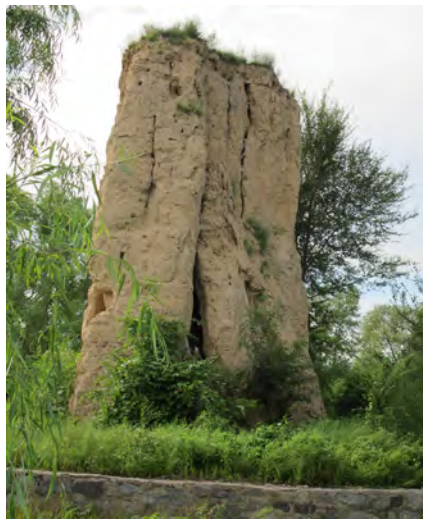
Fig. 4 Fissure deterioration
