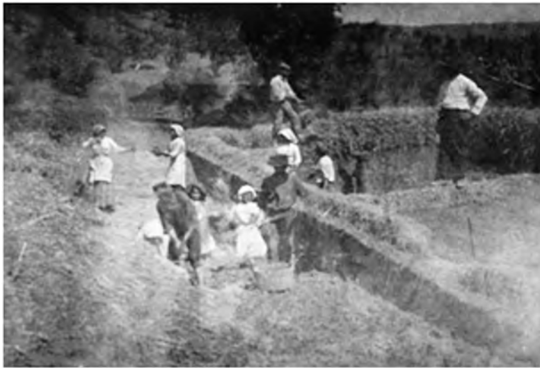
Fig. 3 Historical image of the early XX century: first phase of the earthen construction with the technique of the "massone"
