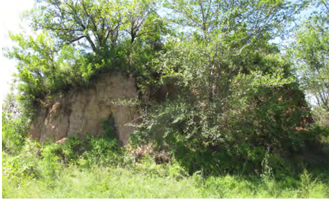
Fig. 7 Biological damage caused by plant growth on earth sites
