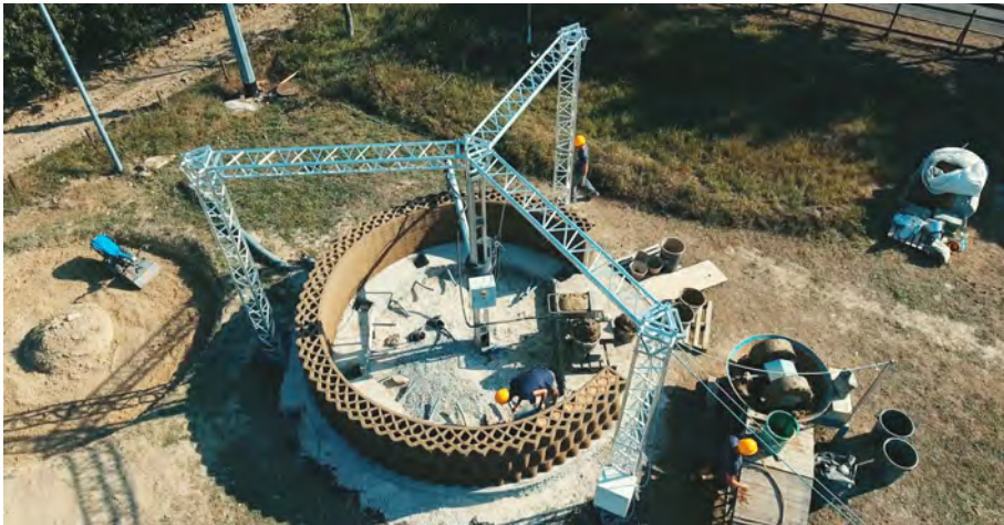
Fig. 1 Crane WASP during the construction of Gaia house, Massa Lombarda, Italy, 2018
