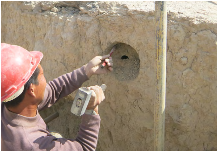
Fig. 3d Enlargement of the hole
