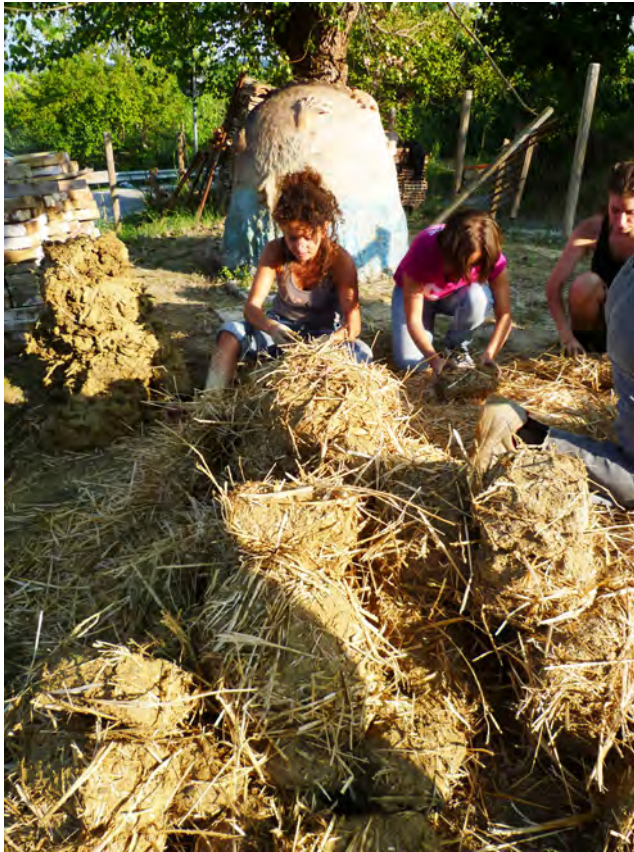
Fig. 4 Restoration site: kneading of the earth for the "massone" technique
