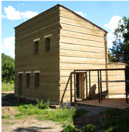
Fig. 3 Rammed earth house in Tuscany (by E. Baglioni, 2013)
