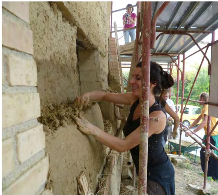
Fig. 8 Casalincontrada (Chieti): Teresa's house, restoration of the walls
