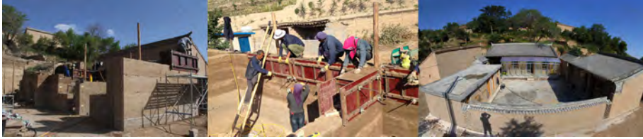
Fig. 9 The first rammed-earth prototype built in the Macha village
