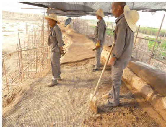
Fig. 9 Capping of the wall against rain erosion
