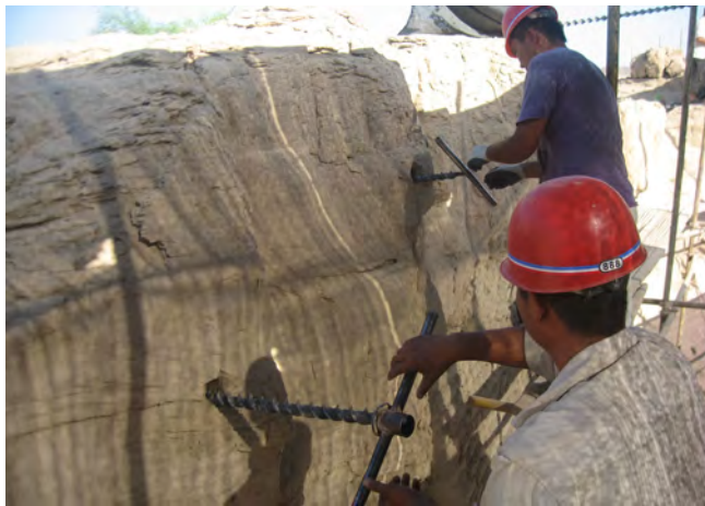
Fig. 3a Artificial drilling
