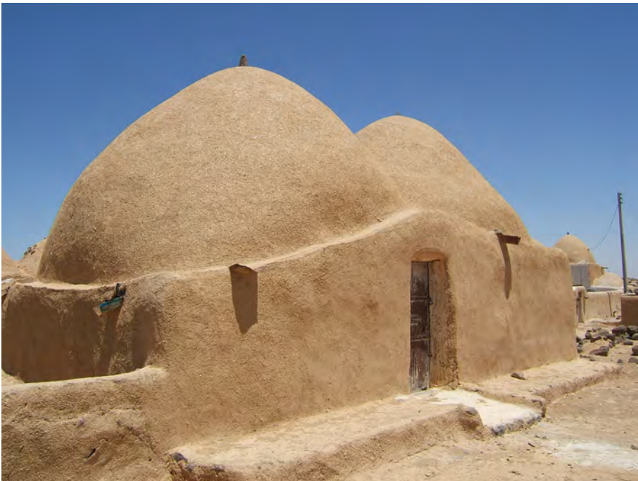
Fig. 2 Syrian corbelled dome house, well maintained
