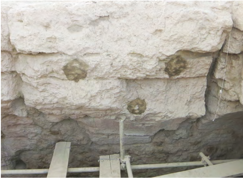
Fig. 3f Sealing the hole
