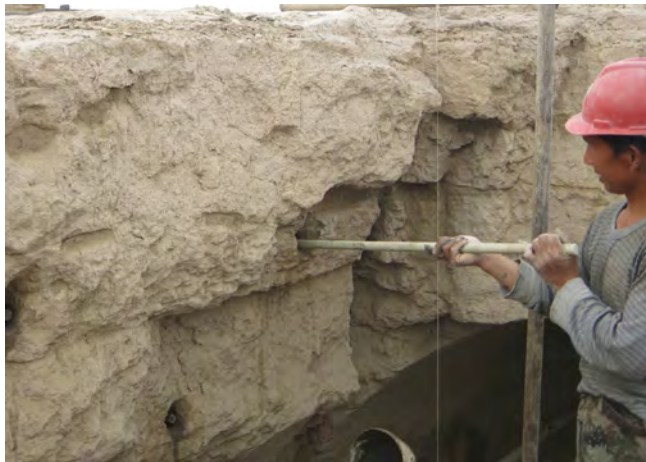
Fig. 3b Bolt installation
