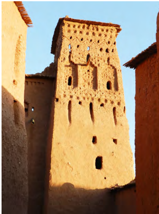
Fig. 6 Earthen building in Ouarazazate (Morocco) (by M. Mattone, 2015)
