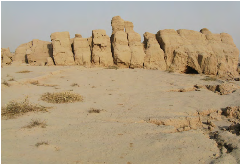
Fig. 4 Fissures on rammed earth walls
