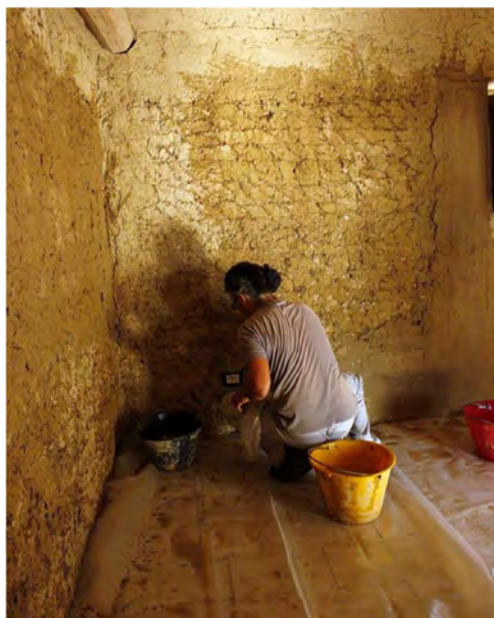
Fig. 9 Casalincontrada (Chieti): Teresa's house, application of earthen plaster
