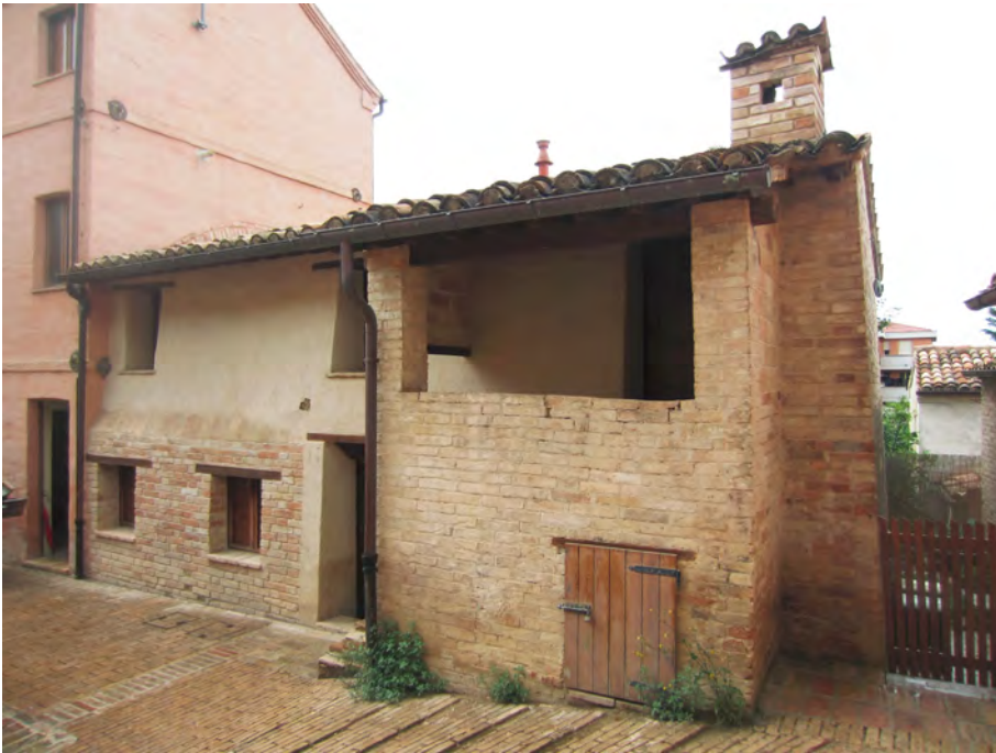
Fig. 1 Exterior of a recovered house in Villa Ficana, Macerata, Italy (Credit by E. Baglioni, 2015)
