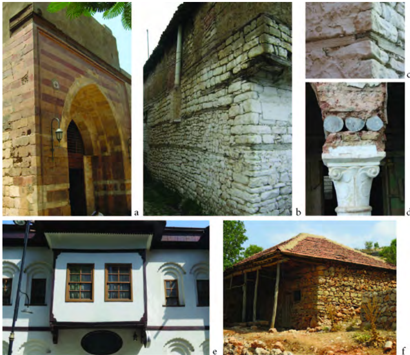
Fig. 4 Examples of anti-seismic and traditional retrofitting techniques making use of timber: a) Bayt es-Suhaymi palace, Cairo, Egypt, XVII century; b) and c) The Kalà of Elbasan, Albania, XV century; d) detail of a capitol of the Dey Palace, Algiers, Algeria, XVI century; e) and f) Malatya, Turkey
