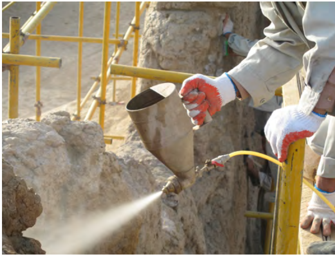
Fig. 10 Application of the consolidating product by spraying
