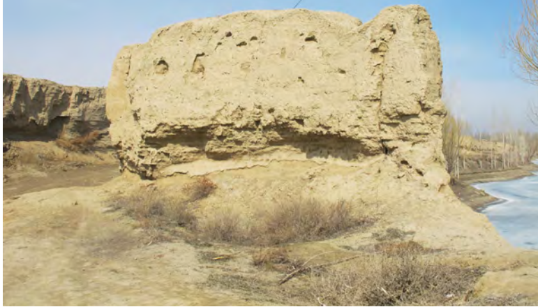
Fig. 3 Erosion deterioration
