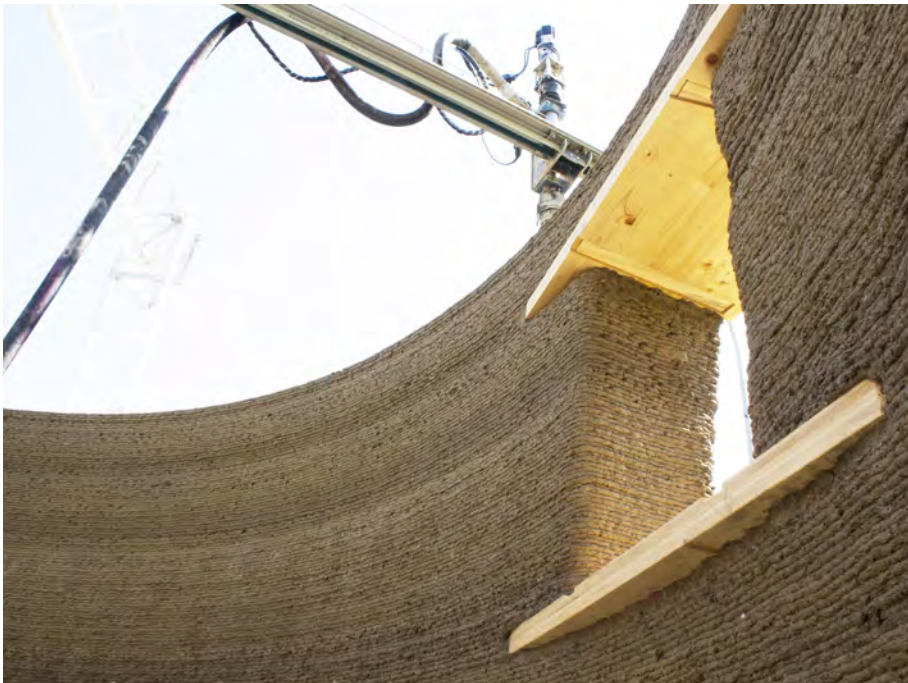
Fig. 4 Earthen mixture in 3D printing process, Gaia house, 2018
