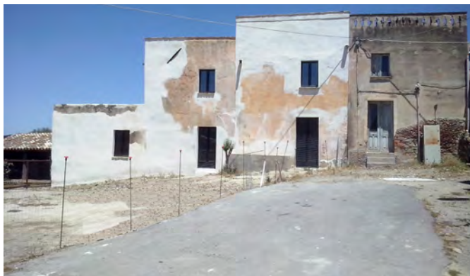
Fig. 7 Medau Palatini, Is Lois, Santadi (SU), exterior of building after restoration (Photo Marco Bianchi)
