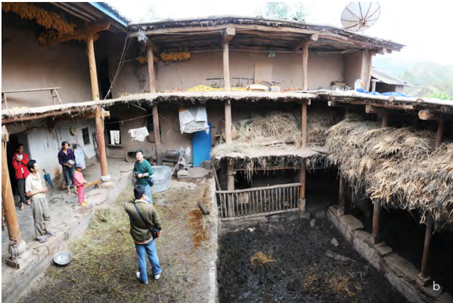
Fig. 6 a-b Local traditional rammed-earth courtyard dwellings and damaged houses after the earthquake
