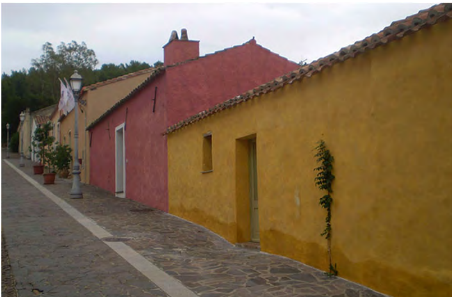
Fig. 5 Sa Domu 'e Pasci, Santadi (SU), exterior of building after restoration (Photo Paolo Pasci)
