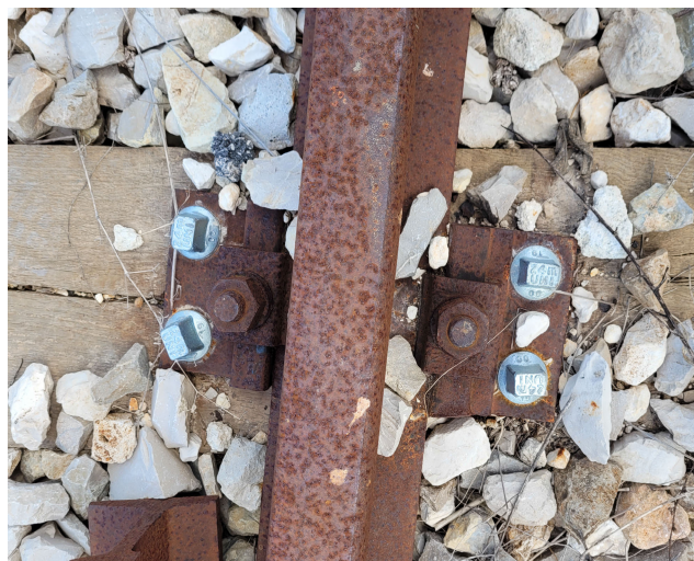
FIGURE 4. Particular of the fastening system, focused on the tie plate.
