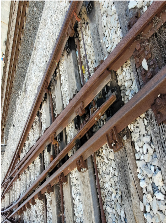
FIGURE 5. An example of railway switch.
