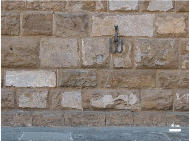
**Figure 5.** Particular of the old nucleus of Palazzo Vecchio (first half of the XIV<sup>th</sup> century). The whitish surface of some Pietraforte ash-lars represent original fractures filled by calcite, which favoured the shaping of the stone.
