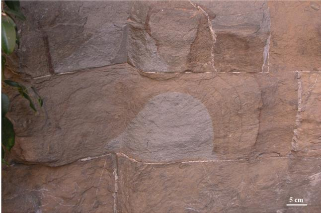
**Figure 11.** Portion of Pietraforte showing inside the original grey colour.
