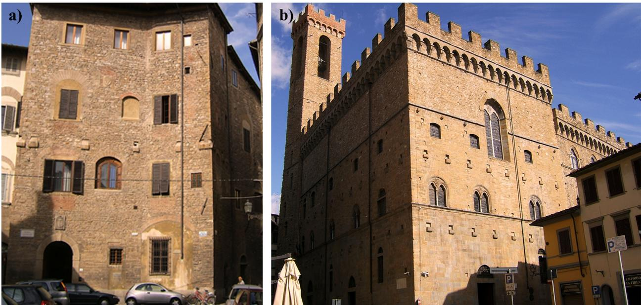
**Figure 6.** a) Tower house made of Pietraforte, in Piazza Peruzzi; b) Palazzo del Bargello, in the image can be seen the first nucleus of the palace (half XIII<sup>th</sup> century), built with partial shaped Pietraforte blocks.
