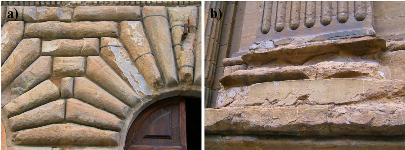
**Figure 14.** (a) *Palazzo Ugucioni (XVI<sup>th</sup> century), example of late Renaissance architecture: fractures and veins filled with calcite representing zones of preferential detachment in the stone blocks;* (b) *Chiesa di San Michele e San Gaetano (XVII<sup>th</sup> century): flaking and intergranular decohesion in presence of plain/convolute laminations.*
