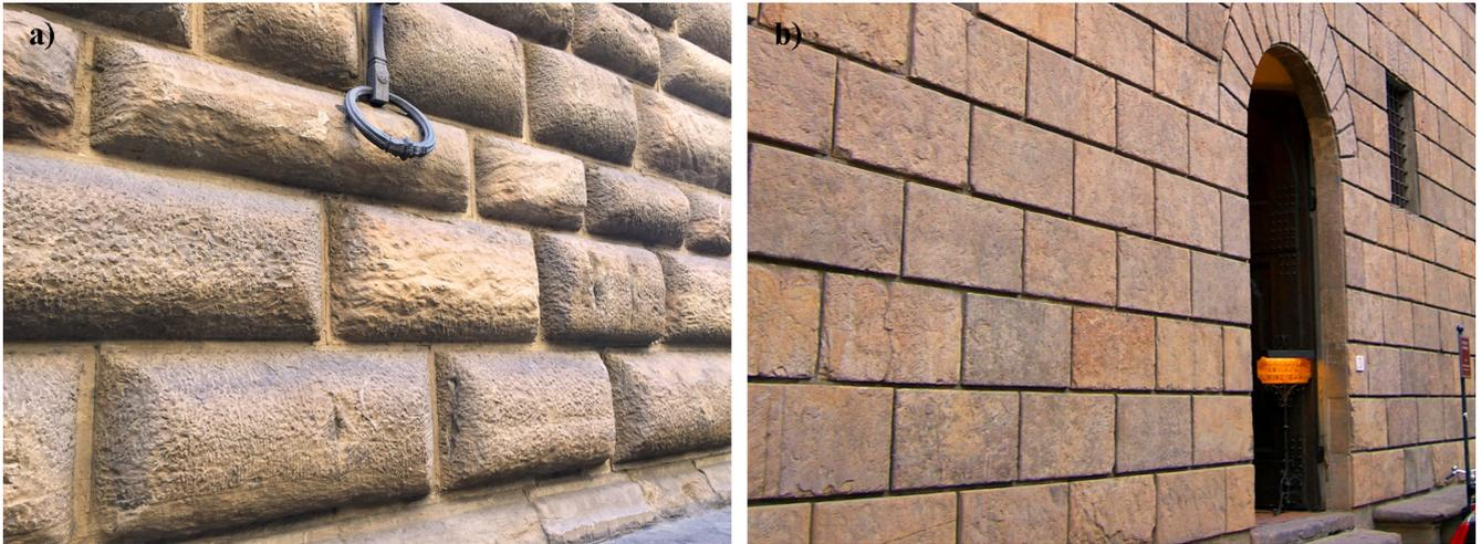
Figure 7. a) Palazzo Strozzi (beginning XVI<sup>th</sup> century), example of late Renaissance architecture, with a façade in Pietraforte quarry-faced ashlars (bugnato rustico); b) Palazzo Antinori (XV<sup>th</sup> century) with the façade in bugnato liscio.
