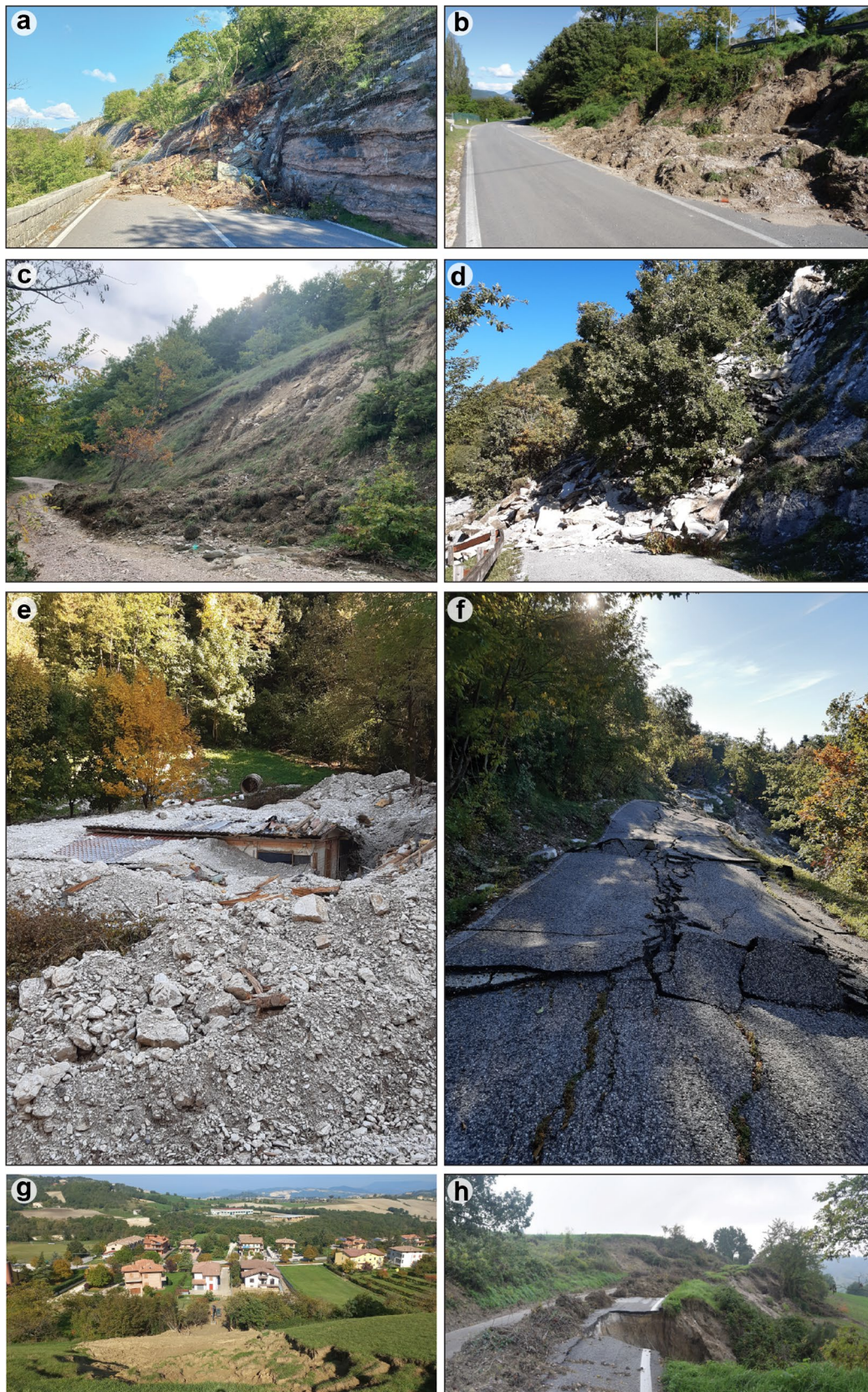
Fig. 5 Examples of landslides that hit roads and structures. a Rock slide on the SS3 national road, Scheggia municipality; b, c, h, g earth slide; d rock fall; e debris flow; f rock slide
