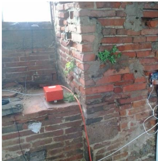
Figure 5. A SARA seismic station installed on the bell chamber.
