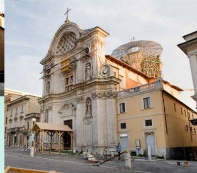
Restoration of Dome
