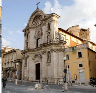
Soon after earthquake Dome ruined
