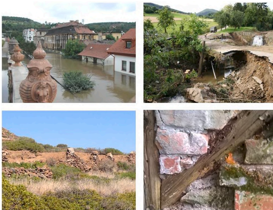
Fig.2. Examples of damages: top left, flooding in historic centre (photo: Drdácý); top right, heavy rain damage in Klingfurth (photo: Austrian Armed Forces, 2009); bottom left, erosion and partial collapse of dry stone walls in the Island of Filicudi, Aeolian Archipelago (photo: Sardella); bottom right, water damage to half-timbered wall (photo: Cacciotti, 2015).
