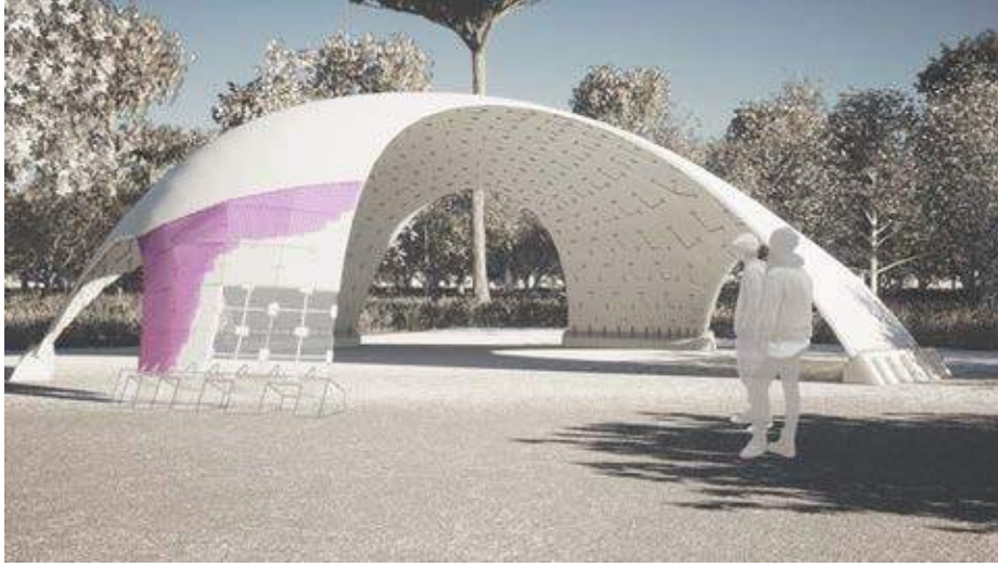
Fig. 1. Conceptual view with technical details of our concrete shell: the shape is segmented into flat tiles that are jointed at the midpoint of the edges and post-tensioned; the outer surface is finished with wire patches and in situ casting.
