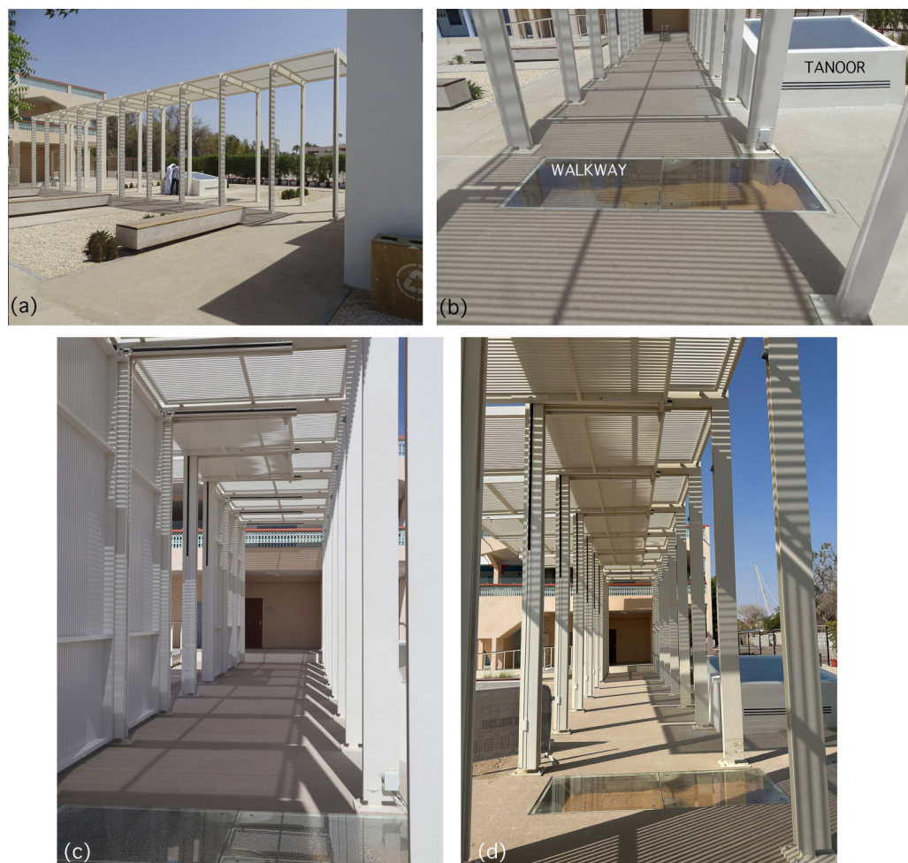
Figure 1. The pergola and the two showcases. (a) Side view of the pergola as it was during the monitoring period, with the family quarters in the background. Small vegetation and a tree are planted in proximity of the pergola. (b) Detail of the glass top of the walkway showcase in the middle of the pergola and the tanoor showcase on the right side. (c) The pergola as it is now, with the operable louvres in vertical position to separate the walkway from the courtyard. (d) The operable louvres in horizontal position, protruding from the ceiling, to connect the eastern and western courtyards. Note that in both the vertical and horizontal positions the shade is partial, part of the solar radiation passing through the gaps between slats.
