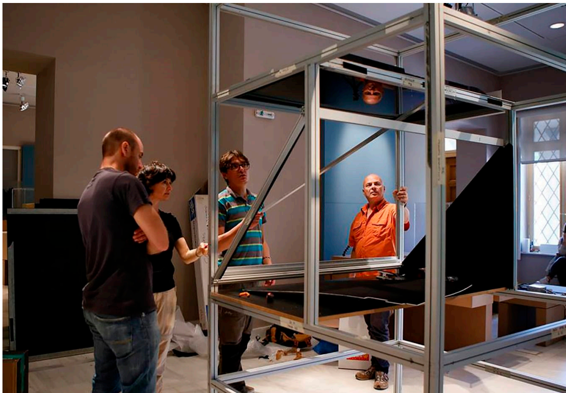
Figure 10. Structure of the showcase in aluminum profiles, a step of the setup.
