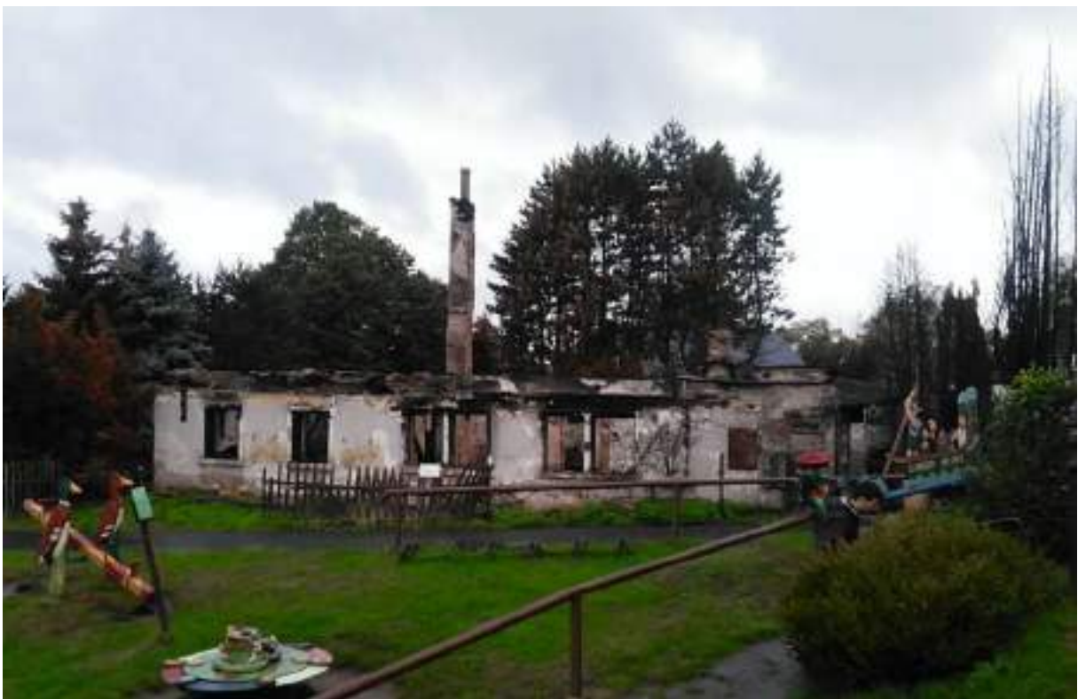
Figure 93. House destroyed by fire in the centre of Mezná. The house was not located close to the main burned area. The burning was likely caused by flying embers that ignited the coniferous garden hedges (right side).
