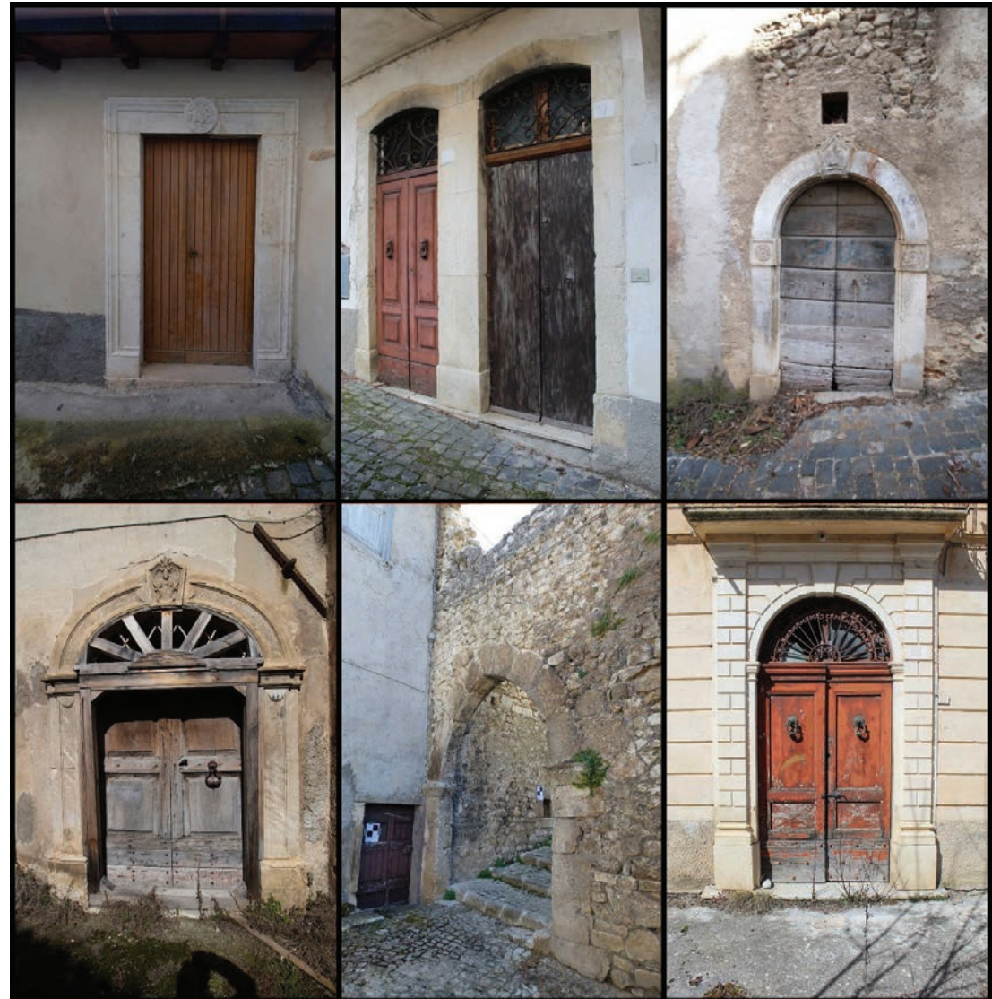
Fig. 5 - Example of portal types identified in the historic centre of Fossa.
