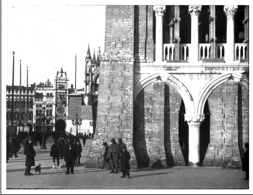
Fig. 4. Venice, the Doge's Palace, detail of the masonry structures reinforcing the arches (Historical Archive of the Navy).
