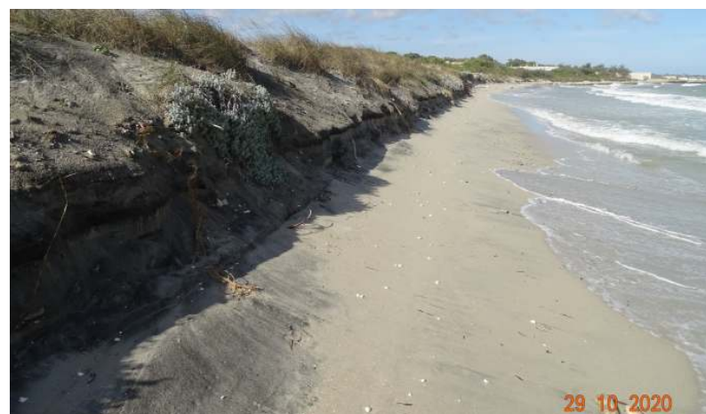
Figure A5. Dune toe erosion due to swash action (northwest sector).
