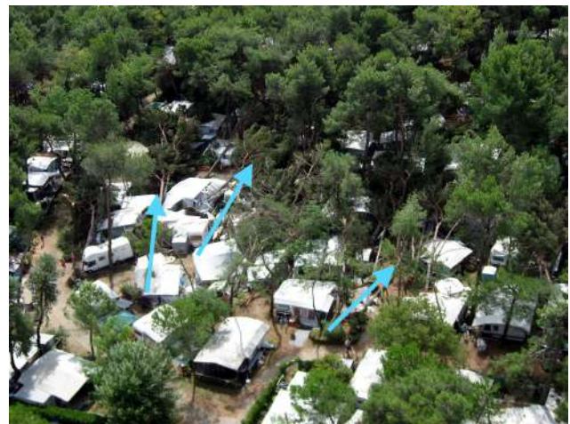
FIGURE 2 Photos of damage reported in the Grado camping site. The parallel trees pulled down suggest linear winds instead of tornadic winds. Arrows indicate the position and direction of fallen trees
