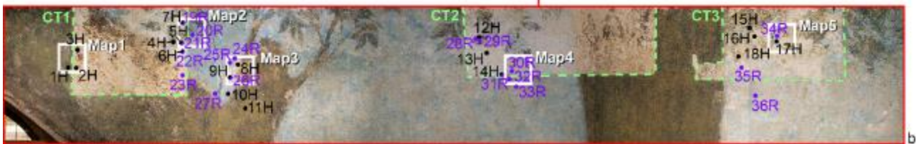
Fig. 1 (a) Scheme of the north-west wall with indication of the analysed area (red rectangle) and the location of the three cleaning tests (CT1-3); (b) digital reconstruction of analysed area with indication of cleaning tests (CT1-3), XRF point measurements (1H-18H), Raman measurements (19R-36R) and XRF maps (Map1-Map5); the digital reconstruction was obtained merging several pictures of the wall. The original pictures can be found in the supplementary material (Figure S1).
