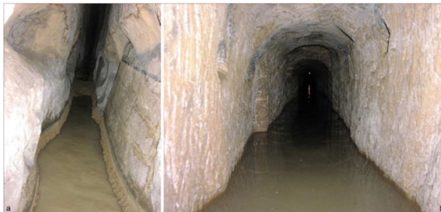
Figure 3. Views of the underground specus explored during speleological survey in Boccaladrona locality: (a) the left wall of the tunnel, reinforced by small blocks of limestone, is evident; (b) a sector of the channel entirely carved in local stone.
