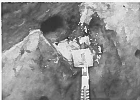
Figure 3. Particular of the ancient whitish adhesion mortar.
