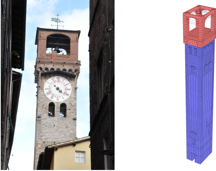
FIG. 7. On the left, a picture of the clock tower in Lucca. On the right, the mesh used for the finite element discretization, where the different materials for the bell chamber and the lower part of the tower are reported in different colors (respectively red and light blue).
