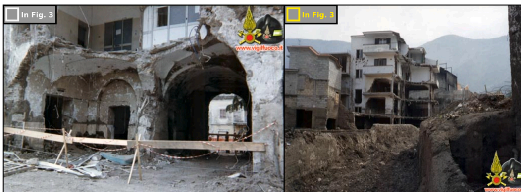
Fig. 4. Photographs showing the collapsed part of the hospital (left), and a building penetrated by mud and debris that overflowed from the abandoned drainage channel (right) (credits: www.vigilfuoco.it ). Location of these buildings is indicated by squares in Fig. 3, according to the corresponding colors here displayed.
