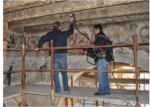
Fig. 6- The surveyed wooden structures (photo by Giovanni Leucci)
