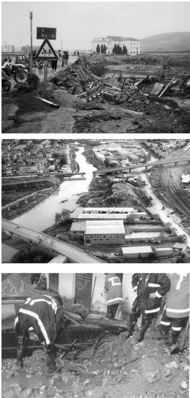
Fig. 17.6 Crotona DHE. Top and middle photos , Crotona town after the flood and a broken bridge. Bottom image : damage in Cosenza province (Cerisano village)
