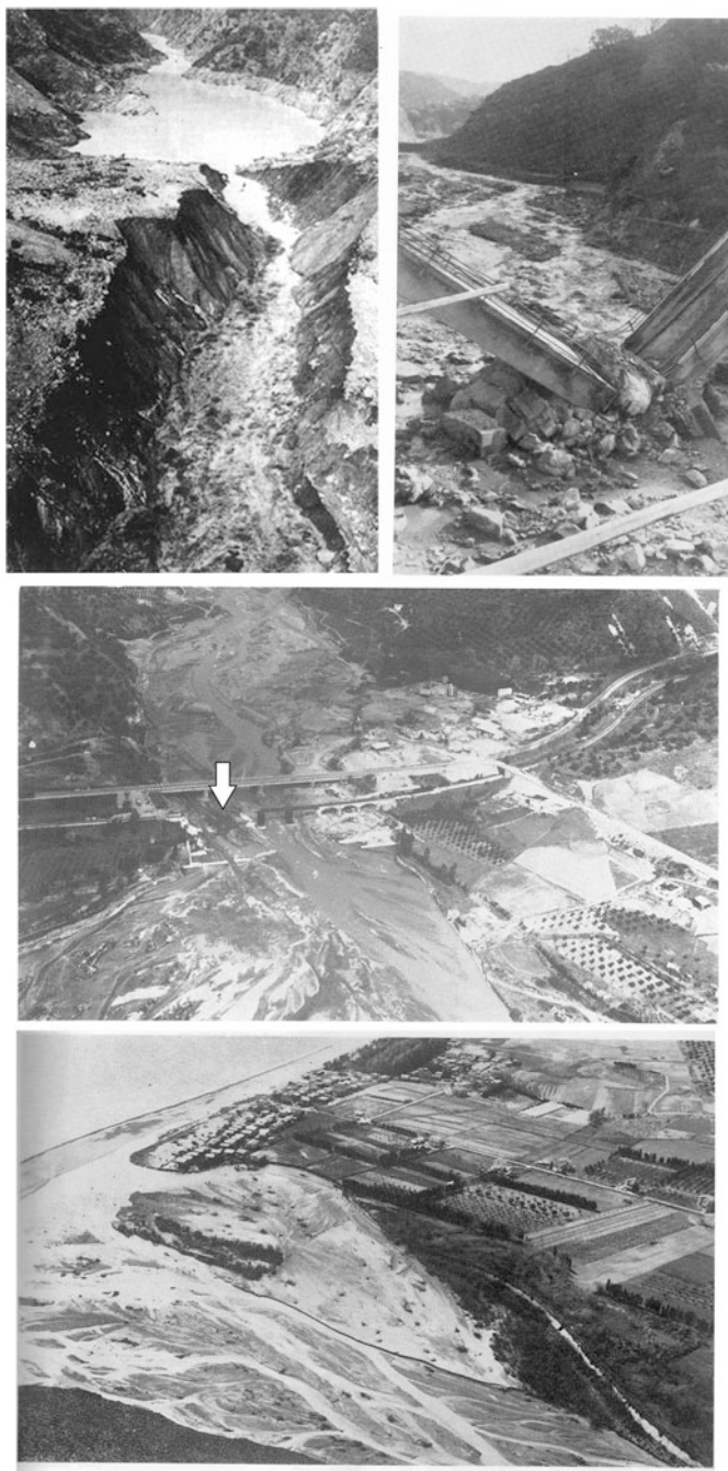
Fig. 17.5 1973 DHE. Top left : the Bonamico landslide lake (Delfino 2004); top right : the bridge on S. Agata river (Reggio C.). Middle image : the railway bridge on Corace river ( white arrow ). Bottom image : the Simeri coastal village threatened by Simeri river) (the last three photos were published in Giangrossi 1973)
