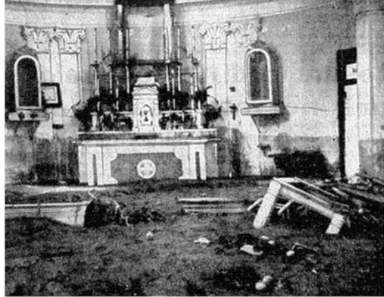
Fig. 17.3 1953 DHE. Top image , the church of Oliveto village (Reggio C.) flooded by a torrent: the priest died near the altar (Photo from the archive of the newspaper La Stampa ). In the middle , some houses of Oliveto village located along a river and damaged by the flood (Photo from the archive of the newspaper L'Unità ). Bottom , the railway damaged by sea storms in Reggio C. province (Photo from the archive of the newspaper La Stampa ).
