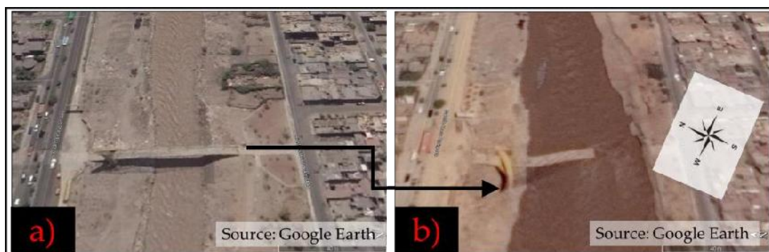
Figure 11. Google Earth imagery (© 2020 Maxar Technologies) acquired on (a) 28/01/2017 and (b) 21/03/2017 showing the Talavera Bridge prior and after the collapse due to the 16/03/2017 flood event, respectively. In (b) the increase of the water flow of the Rímac River is apparent.
