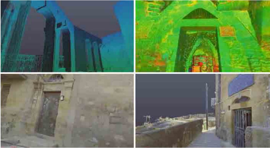
Fig. 3. 3D laser scanning for Qaqish house (Interior & exterior features) (Source: Authors)
